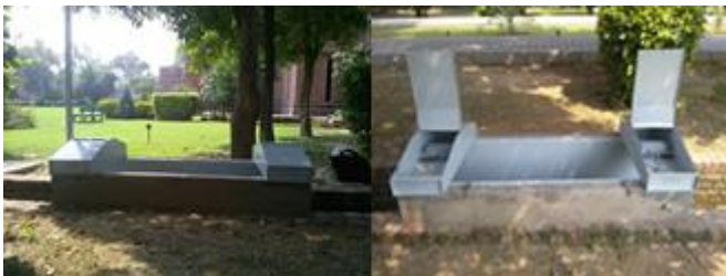
Fig. 2. Smart water meter installation at LUMS campus on a steel flume before being inserted in a drainage channel [10]
