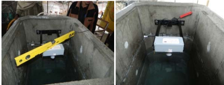
Figure 4.1(b): Instrument installations, alignment and leveling. (c): Installed Unit
