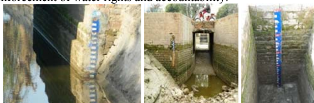
Figure 1(a): Examples of manual gauge readout settings for pansal nawisi by Punjab Irrigation Department in Hakra Branch, Bahawalnagar. The water levels are converted to flow using a rating curve derived from channel geometry.
