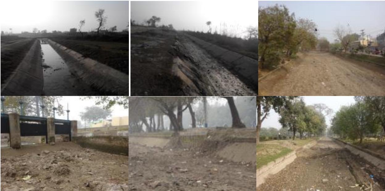
**Figure 1.** Examples of irrigation channels in Lahore district (Punjab, Pakistan) during annual inspection for siltation. A small channel with paved banks (Top Left). A small silted channel identified for cleaning (Top Center). A large distributary canal before silt cleaning (Top Left). Close view of siltation and bank damage (Bottom). (Photographs taken in January 2016).
