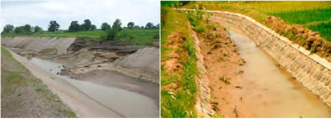
Fig. 1. Examples of bank deterioration (left) and siltation (right) in irrigation canals.
